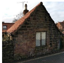
No 7: Nailmakers Cottage & Workshop William St.
